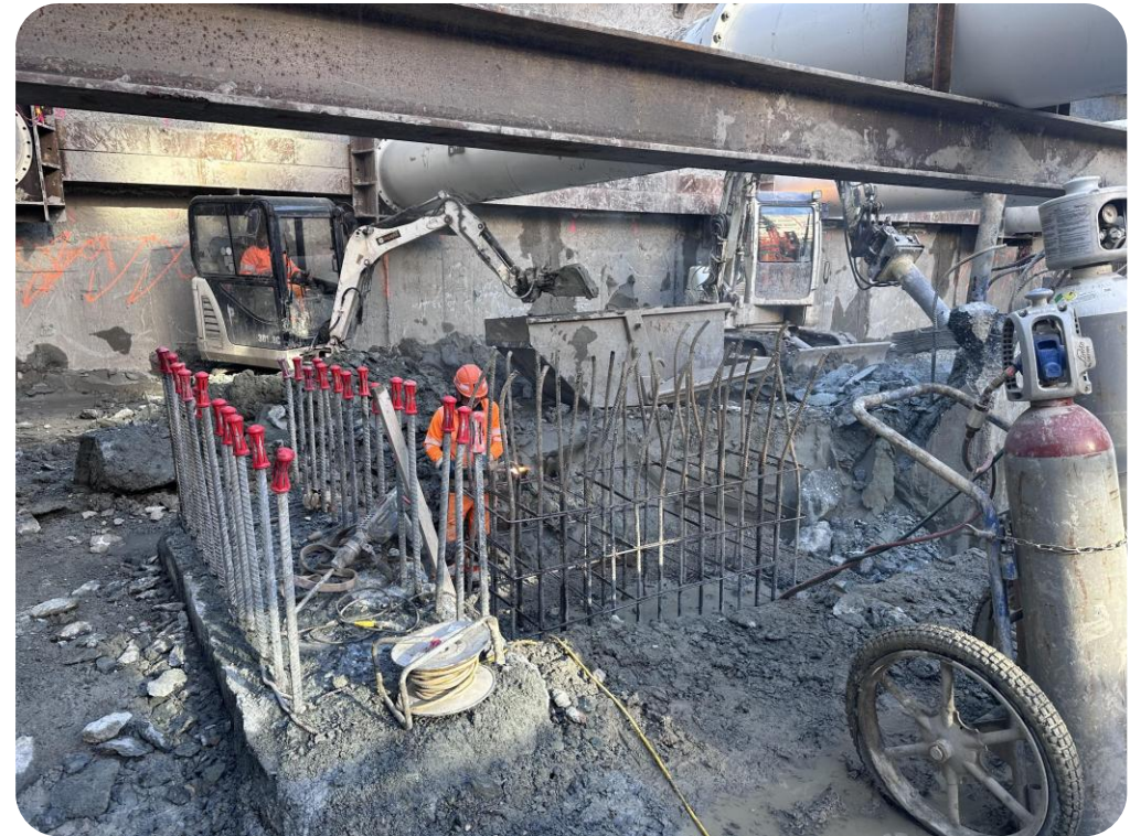
Barrette with exposed reinforcement after trimming to the cut-off level
